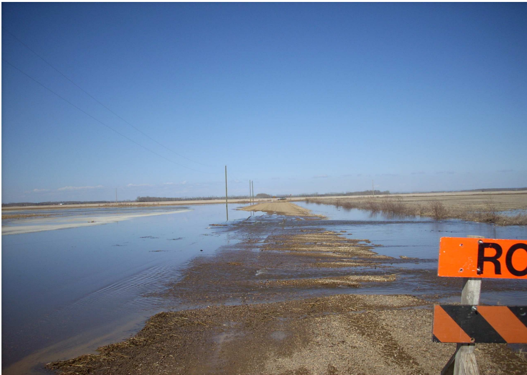
RR 14-0 Looking North
