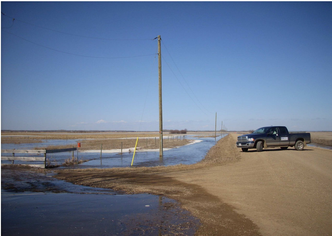
RR 14-0 Looking North
