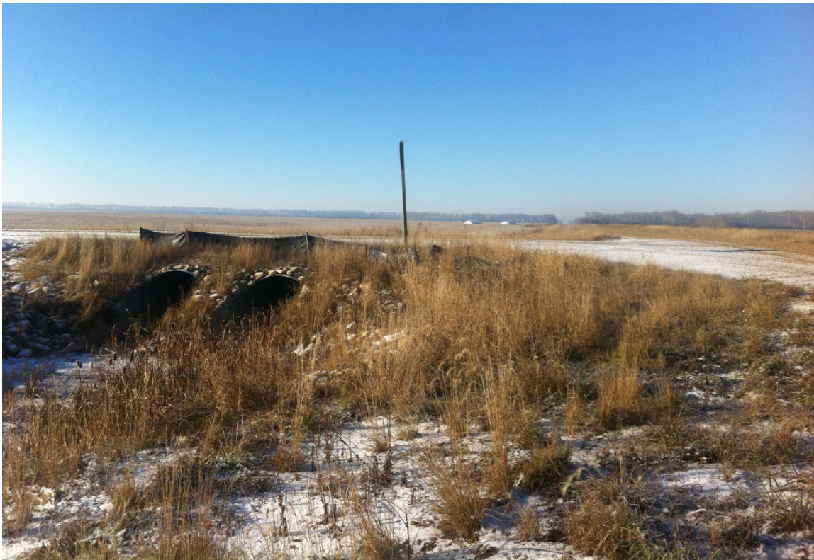
32 - AJA Drainage @ RR 13-4 - Looking West
