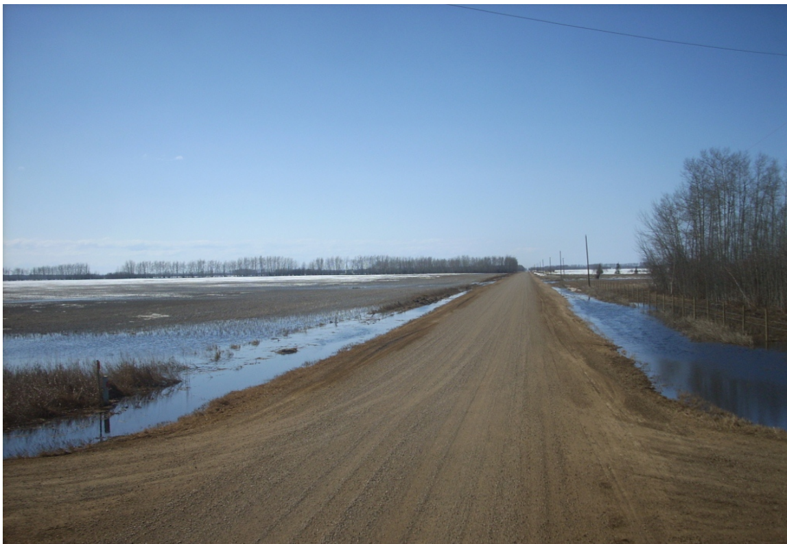
18 - TR 107-2 and RR 12-4 - Looking West (April 2014)
