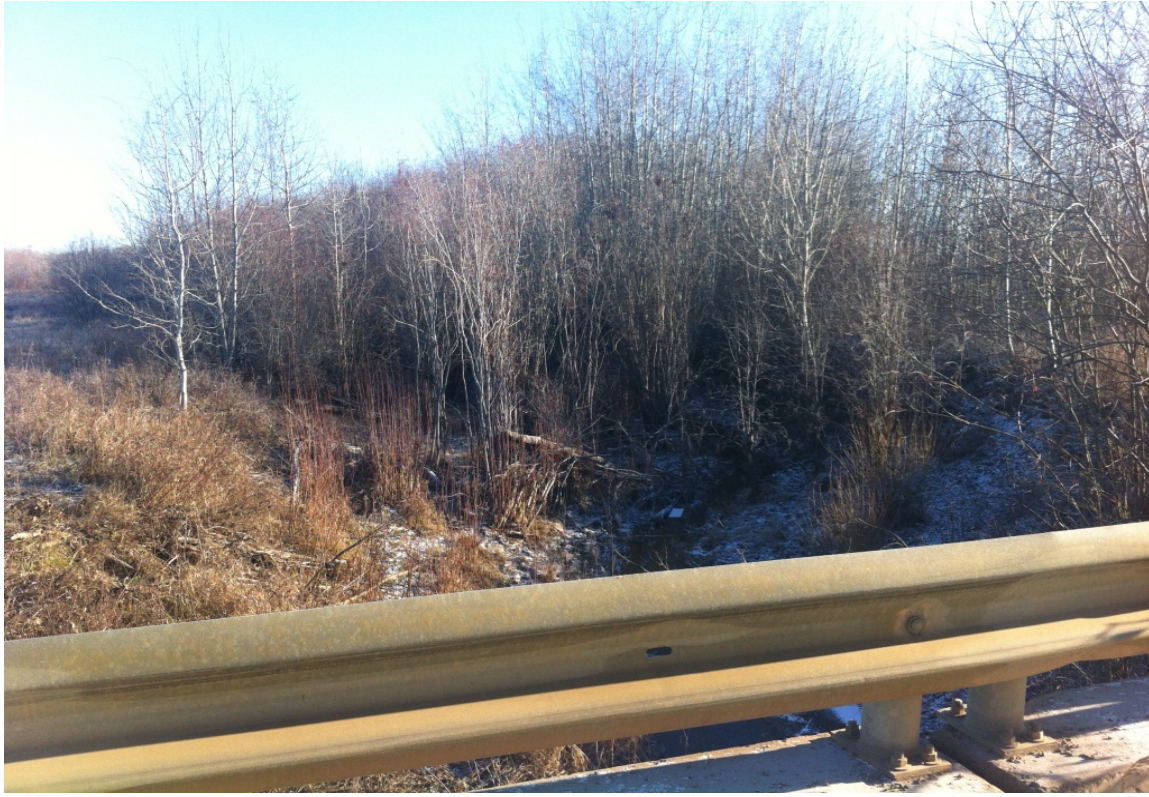
45 - Teepee Creek Drainage @ RR 14-2 - Looking East
