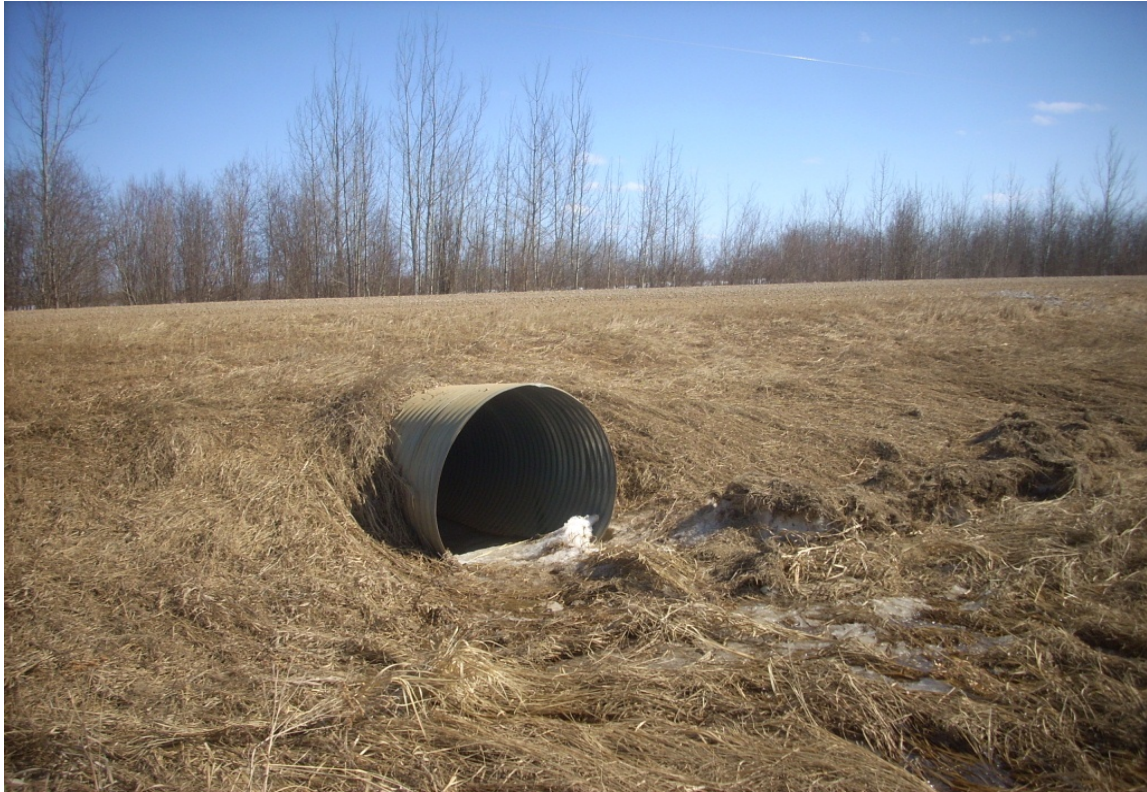
27 - La Crete East Line 1 @ RR 13-1 - 1000 CSP Outlet (April 2014)
