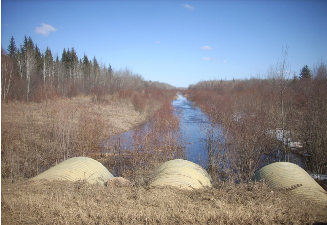
41 - Wilson Prairie Drainage @ RR13-4 - Looking West (April 2014)
