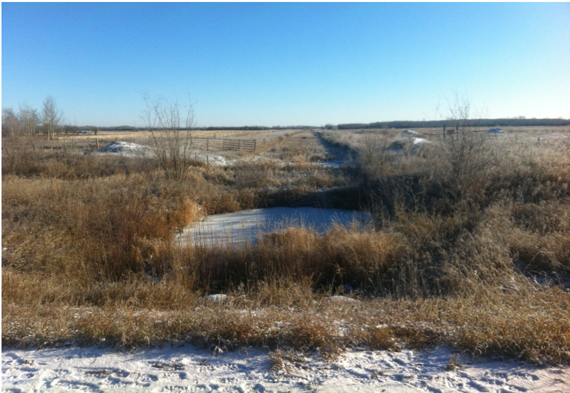
26 - La Crete East Line 1 @ RR 13-1 - Looking East
