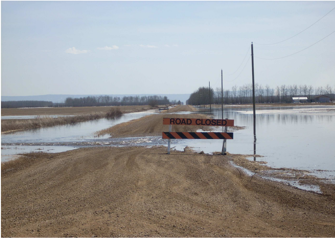
Twp 107-0 and RR14-0 Looking South
