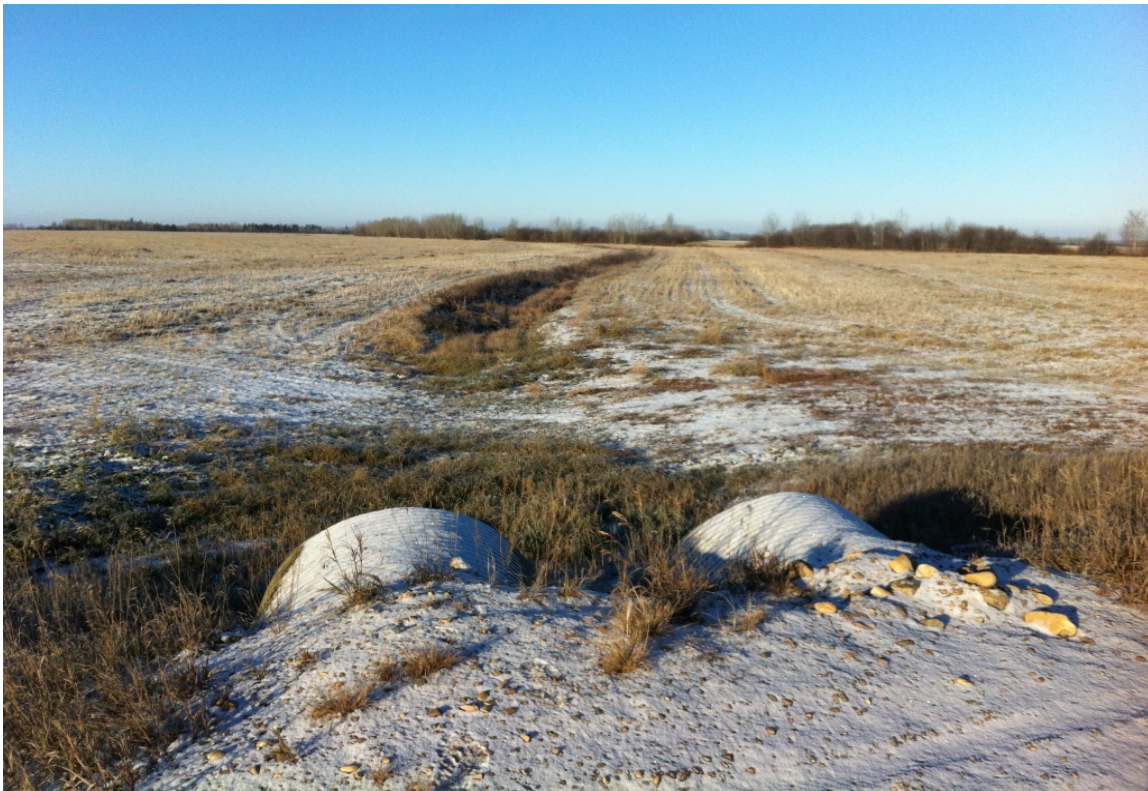
08 - Bear River North Drainage Line 4 @ RR 12-3 - Looking West
