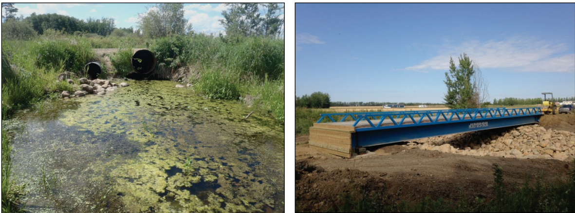
Figure 7-13 Left: Old low level crossing. Right: New temporary portable oilfield bridge.
