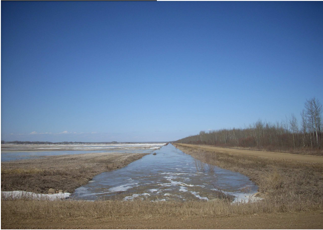
Twp 107-0 Looking West
