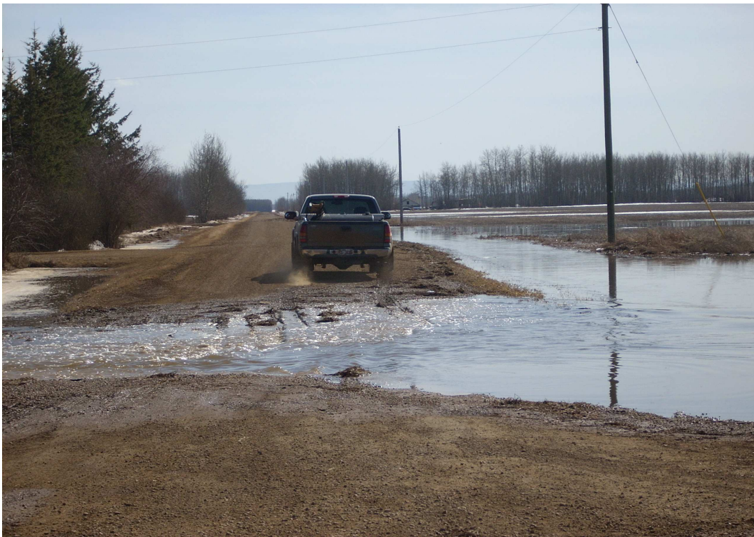
Twp 107-0 and RR14-1 Looking South
