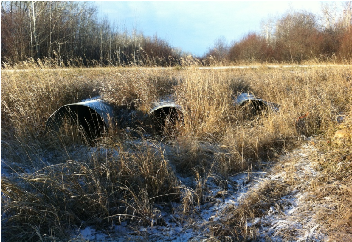
12 - Bear River North Drainage Line 4 @ RR 12-1 - Culverts
