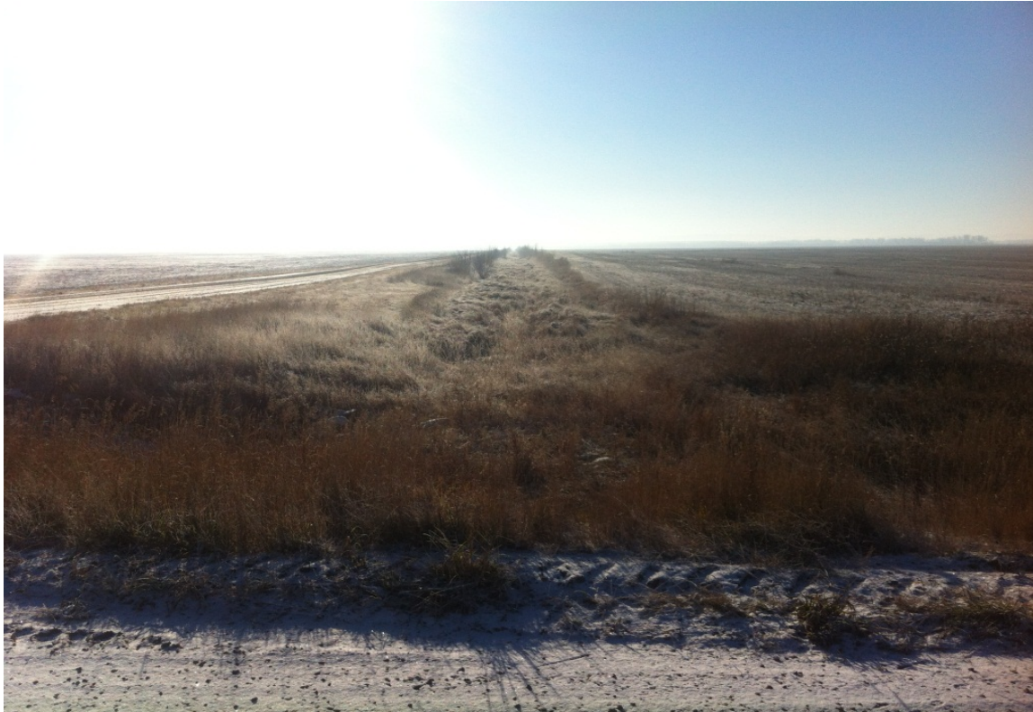
35 - AJA Drainage @ RR 13-4 - Looking South
