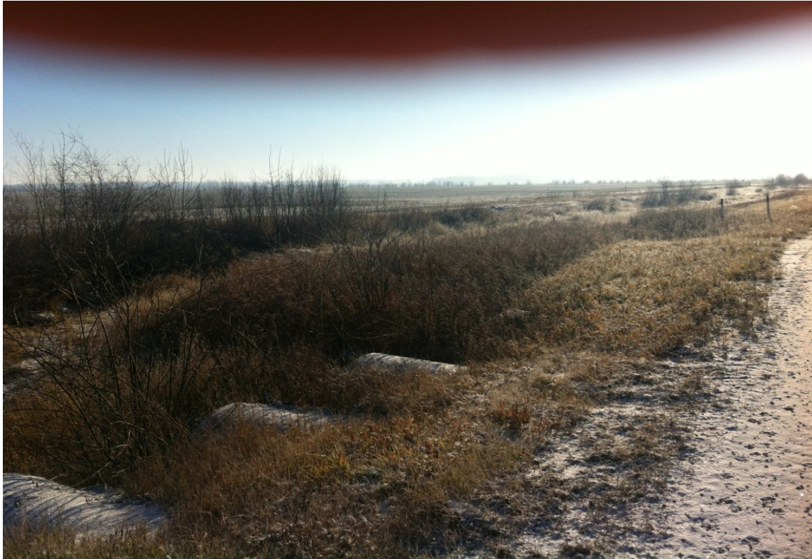
29 - La Crete East Ditch @ RR 14-0 - Looking South
