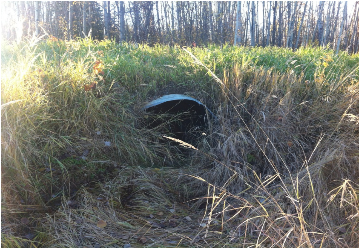
58 - Tributary to Steephill Ck @ RR 16-1 - Culvert
