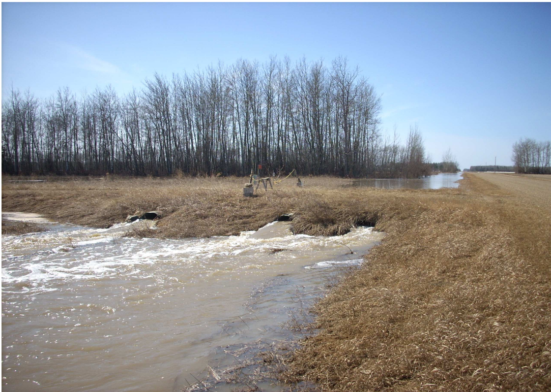
Twp 106-4 Looking West
