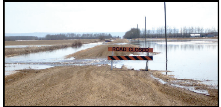
Figure 5-1 Flooding over RR 141 at TR 1070 (2008)
