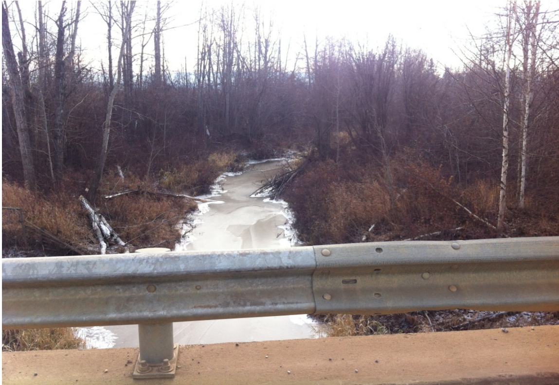
67 - Tributary @ TR 105-0 - BF 76506 - Looking South
