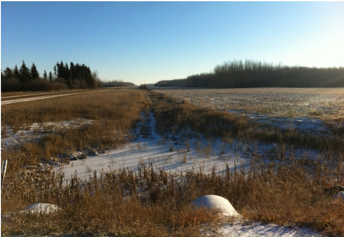
02 - Bear River North Drainage Line 4 @ RR 13-1 - Culverts Across 13-1
