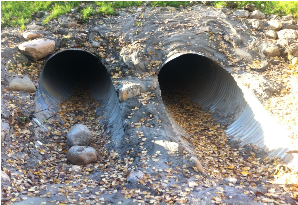
60 - Tributary to Steephill Ck @ RR 16-1A - Culvert
