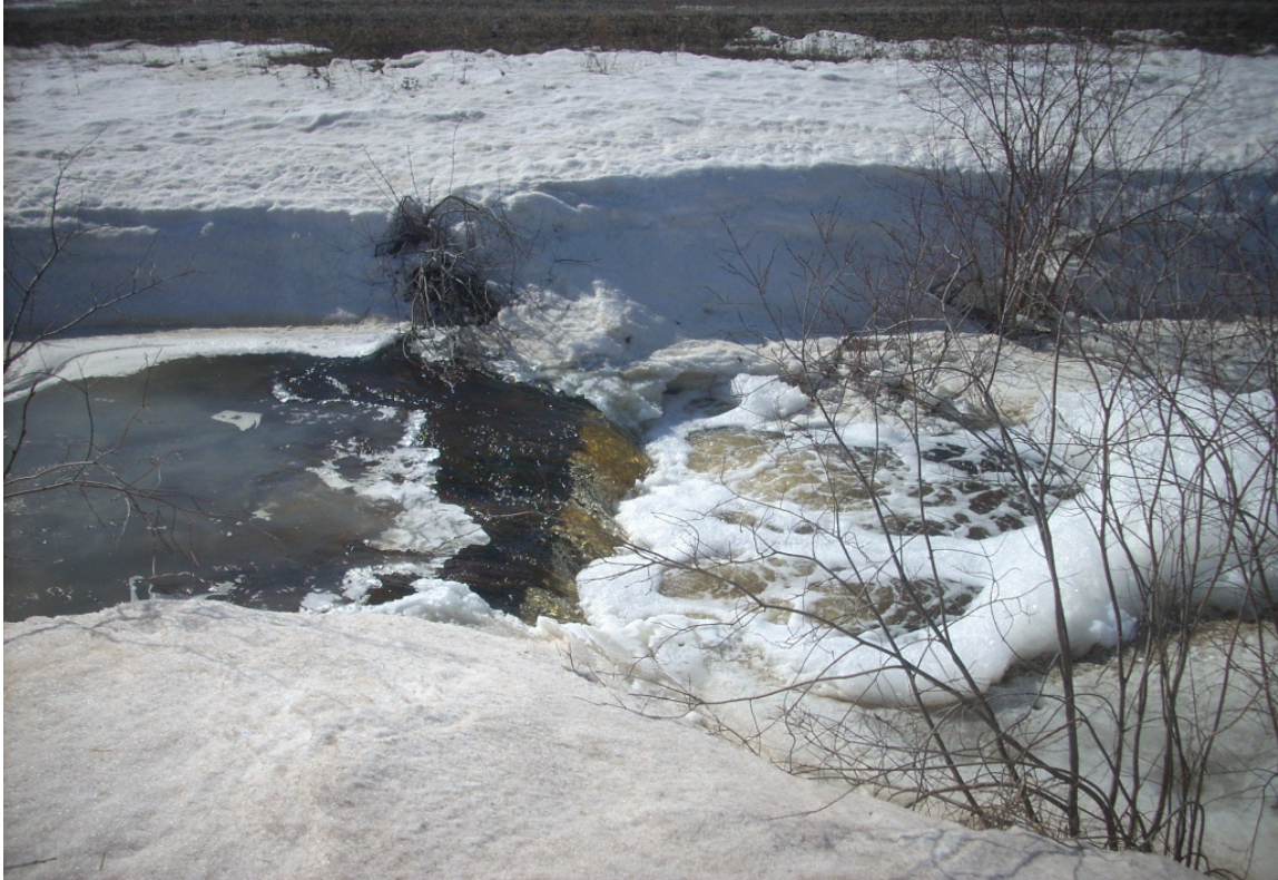
31 - La Crete East @ RR13-4 - Drop structure (April 2014)
