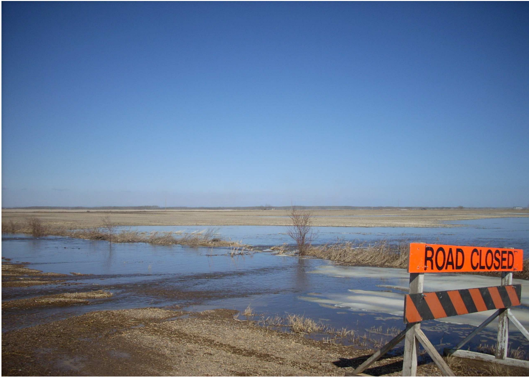
RR14-0 Looking North East
