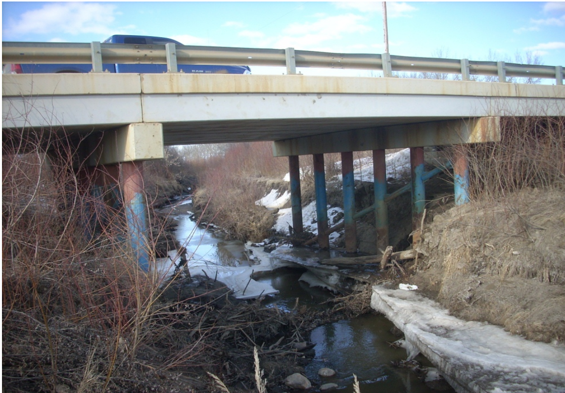
81 - Bear River at TR 105-0 - BF 79552 - Looking North
