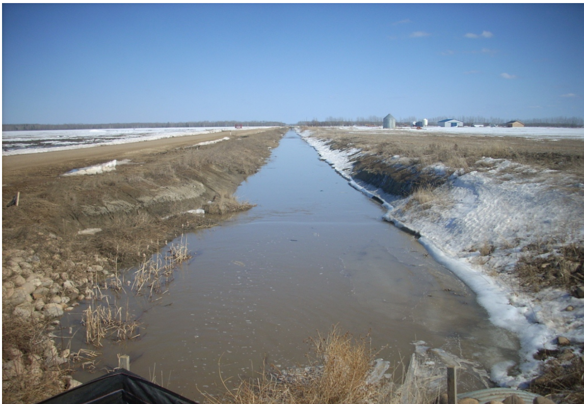
36 - AJA Drainage @ RR 13-2 - Looking East (April 2014)
