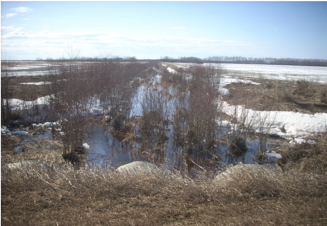
40 - Wilson Prairie Drainage @ RR 14-0 - Looking West (April 2014)
