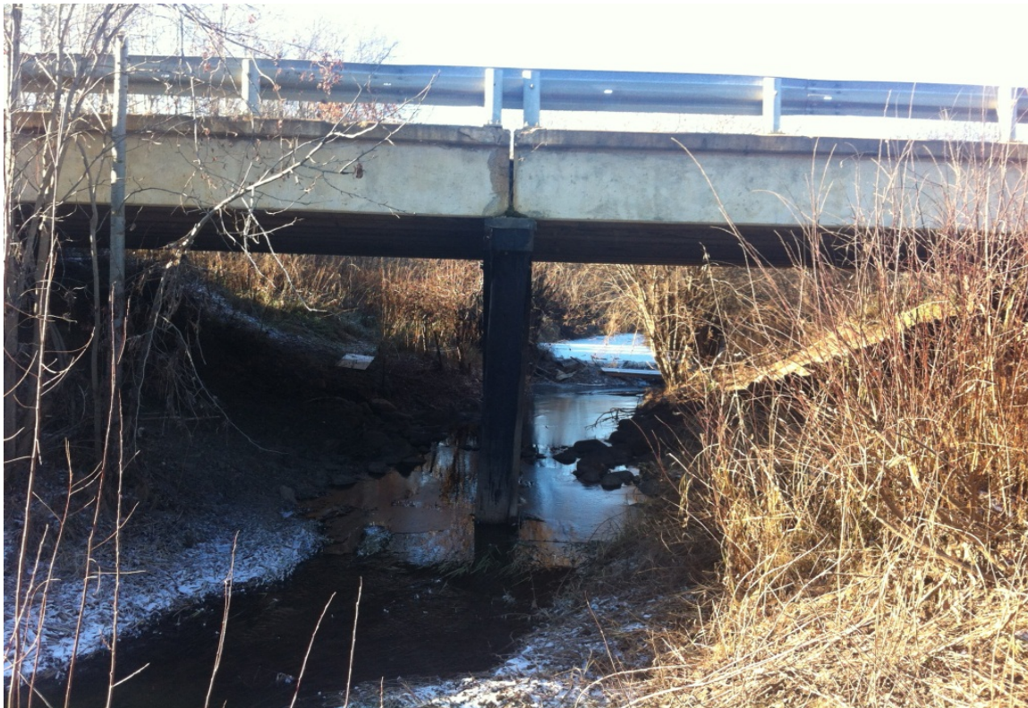
46 - Teepee Creek Drainage @ RR 14-2 - BF 81336
