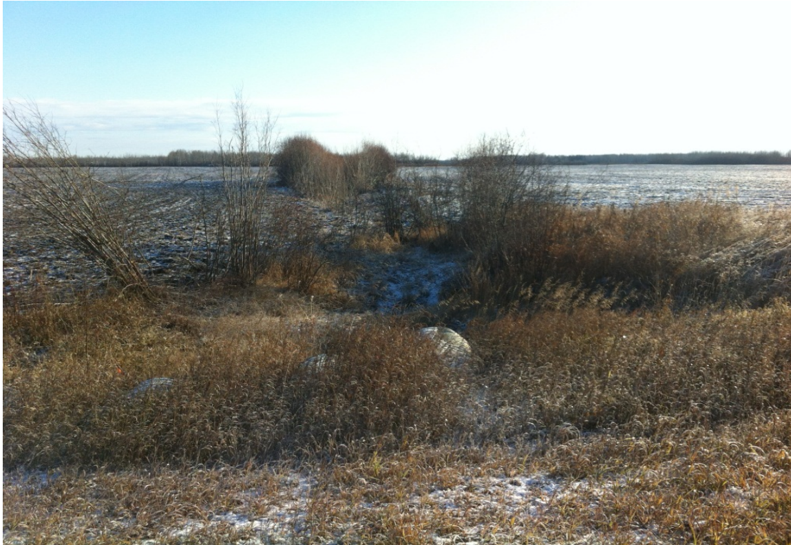
11 - Bear River North Drainage Line 4 @ RR 12-1 - Looking East
