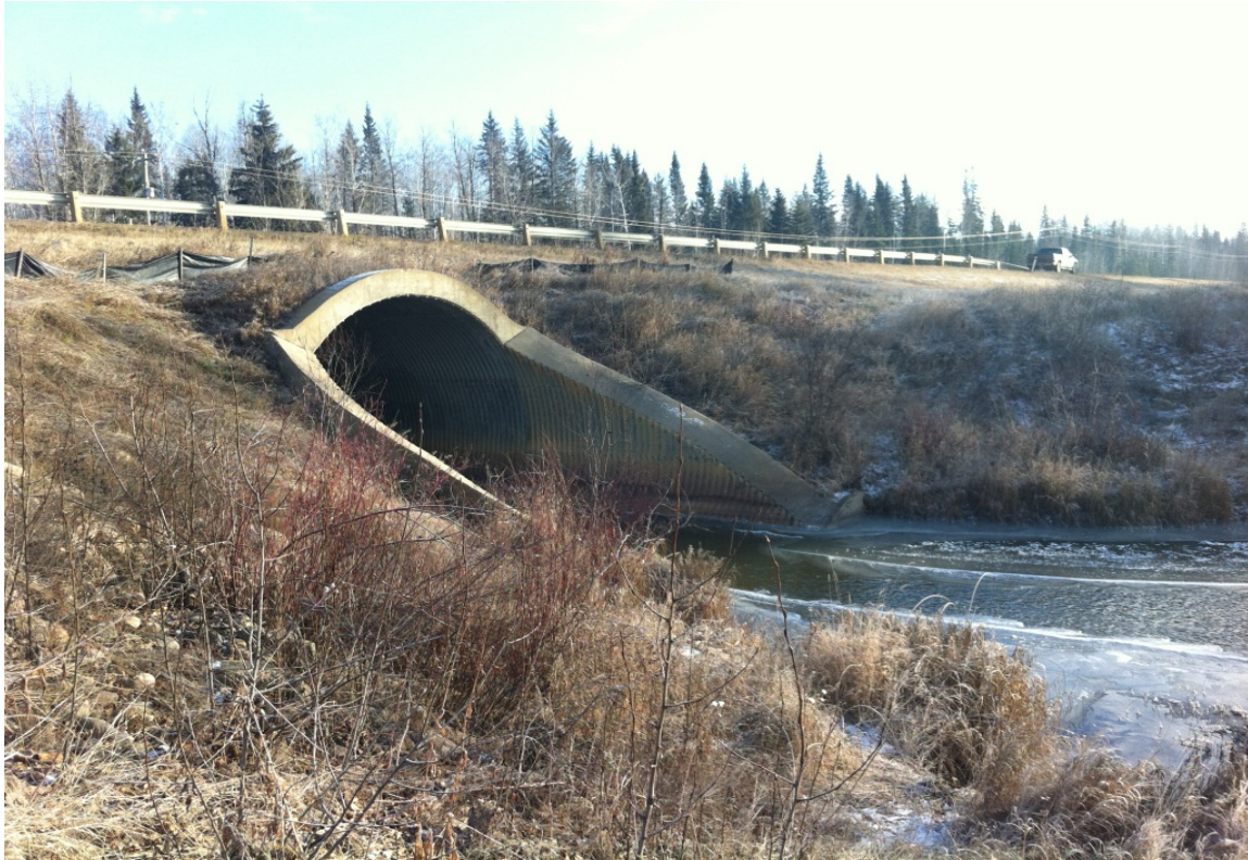
95 - Jackpine Creek @ Hwy 88 - BF 78195 - Culvert Inlet
