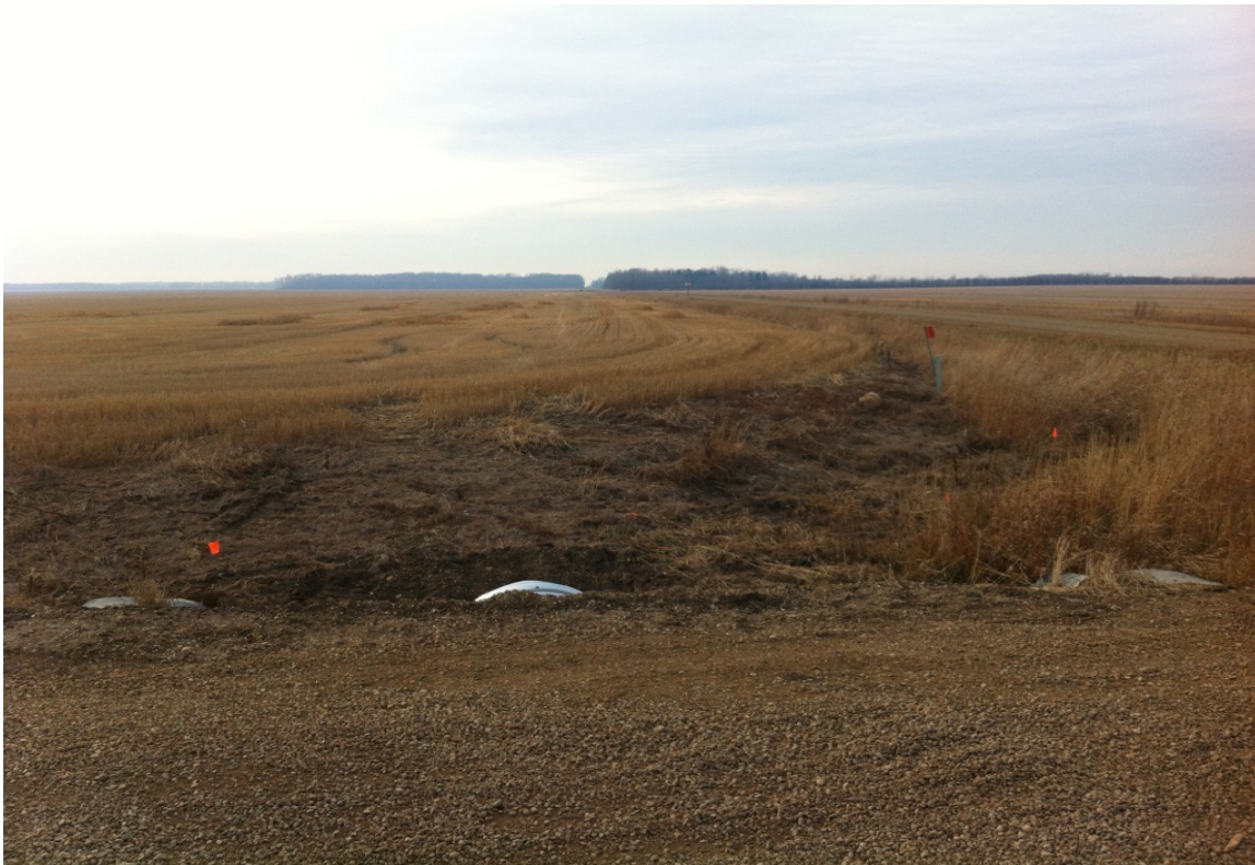
64 - Ditch @ TR 104-4 and RR 14-3 - Looking West
