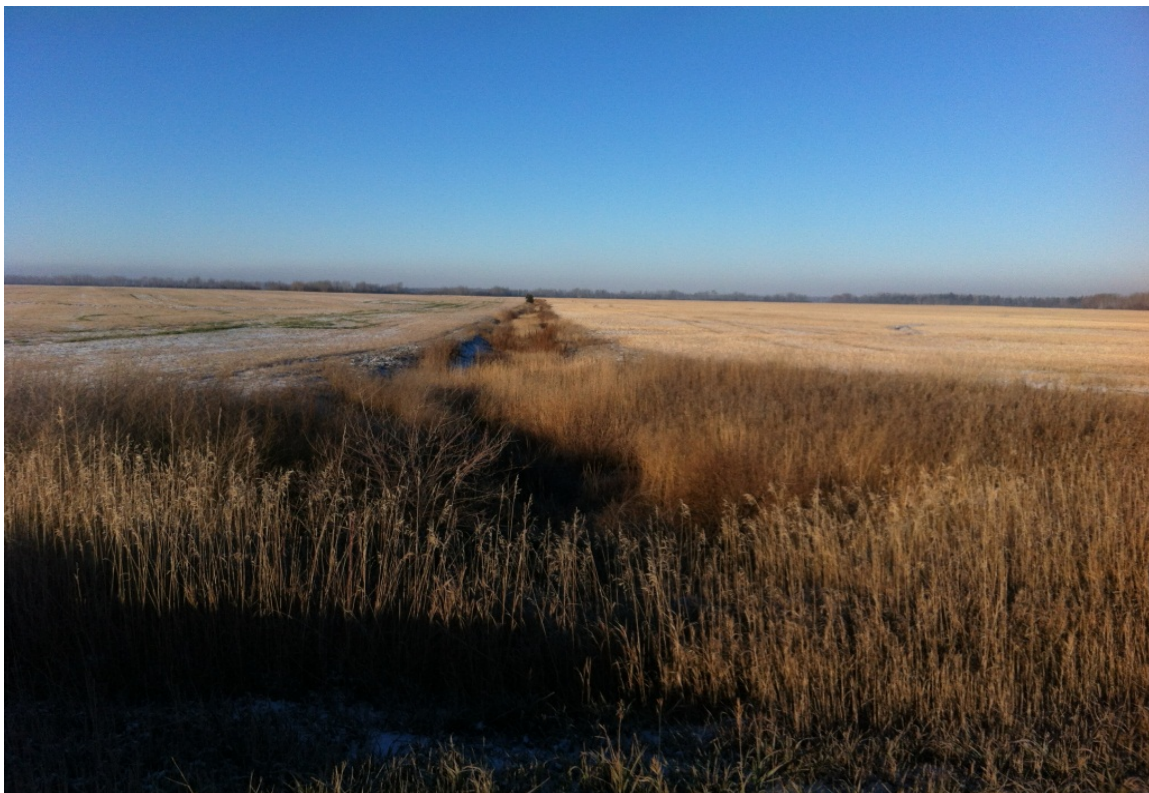
06 - Bear River North Drainage Line 4 @ RR 12-3 - Looking West
