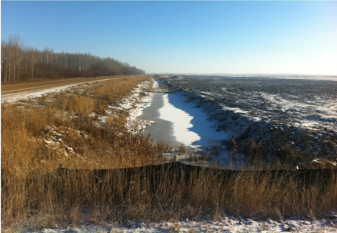
33 - AJA Drainage @ RR 13-4 - Looking East
