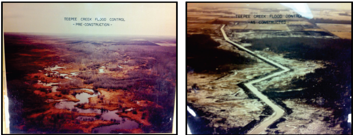
Figure 4-7 Pre-construction (left) and Post-construction (right) photos for the Teepee Creek Flood Control drainage project.
