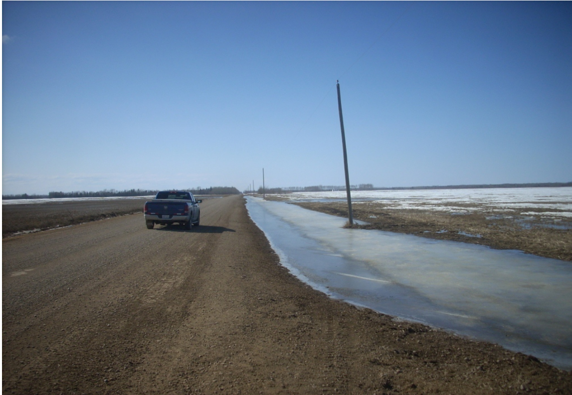
15 - Bear River North Drainage Line 1 @ TR 107-2 - North Ditch Looking East (April 2014)
