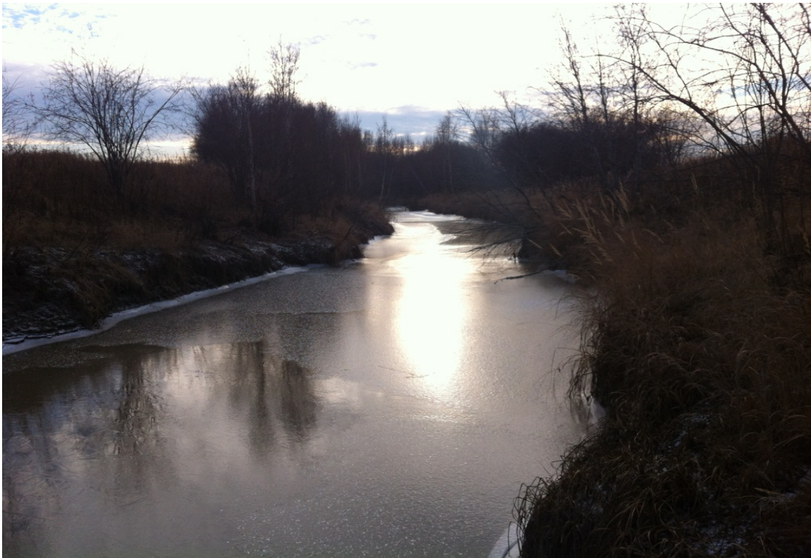
78 - Bear River South of TR 105-0 - Drop Structure - Looking South
