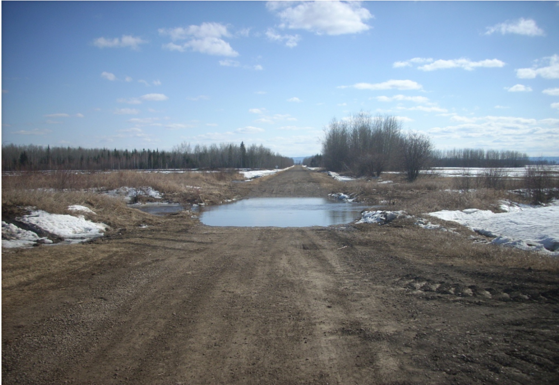
49 - Teepee Creek Drainage @ RR 14-0 - Looking South (April 2014)
