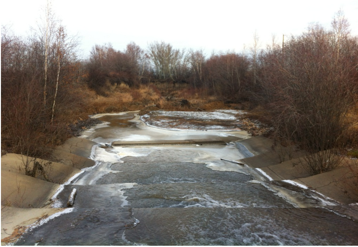
77 - Bear River South of TR 105-0 - Drop Structure - Looking North
