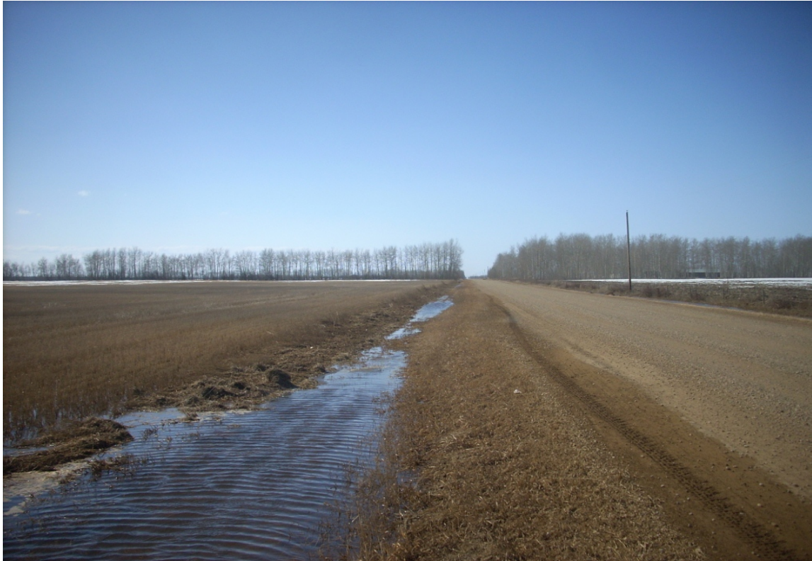
23 - TR107-2 and RR12-1 - South Ditch Looking West (April 2014)
