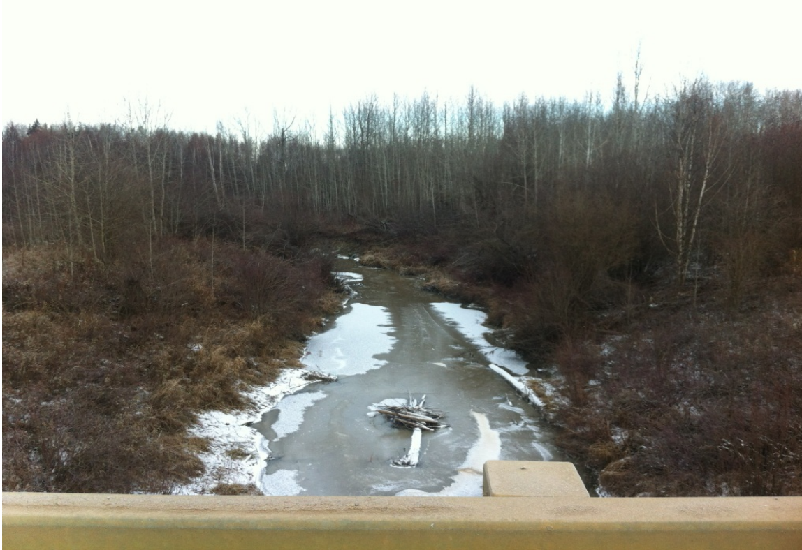
89 - Bear River @ TR 106-6 - BF 80939 - Looking North
