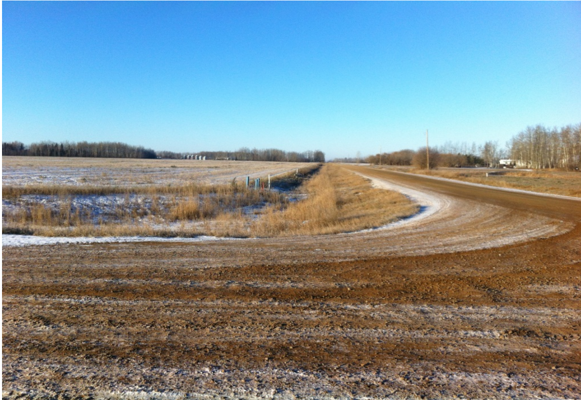
03 - Bear River North Drainage Line 4 @ RR 13-1 - Looking West
