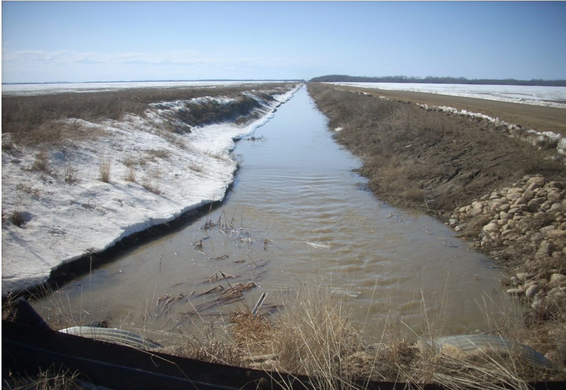
37 - AJA Drainage @ RR 13-2 - Looking West (April 2014)
