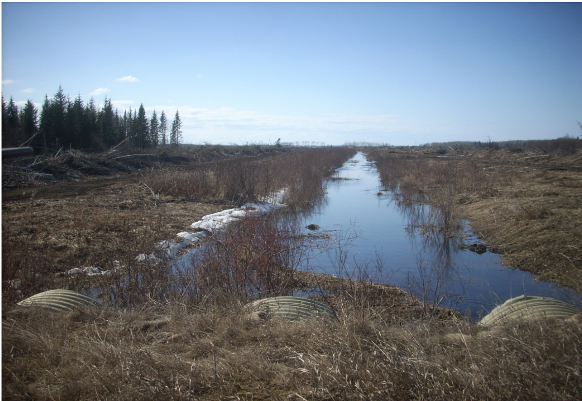
42 - Wilson Prairie Drainage @ RR13-4 - Looking East (April 2014)
